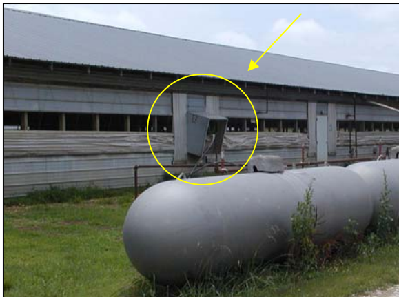
Figure 13: Exhaust fan used for cross-flow ventilation
