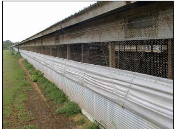
Figure 12: Close-up of plastic drop-curtain (in half-open position)
