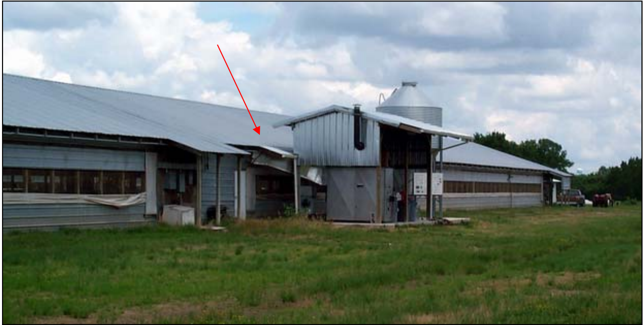
Figure A.1.2: View of furnace and poultry house from the Southeast
