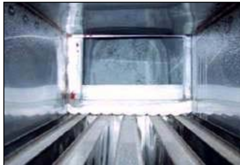
Figure A.4.3: Inside view of air-to-air heat exchanger (foreground) and heat deflector shield (background)
