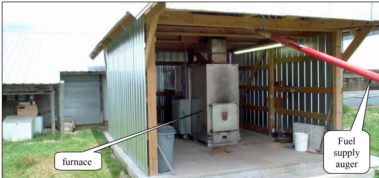
Figure 4: Dobson system installed at UA
